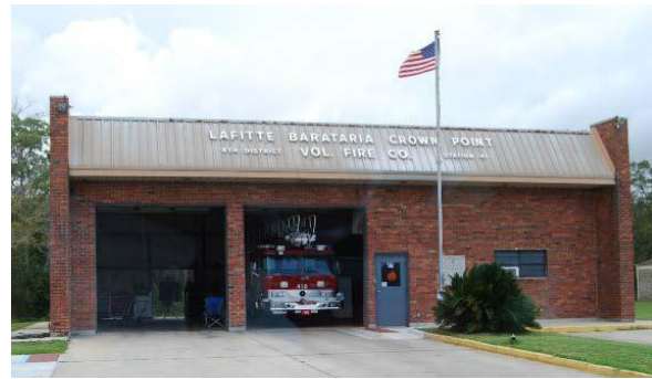
Image #2: Station 41 located at 4176 Privateer Boulevard in Barataria
