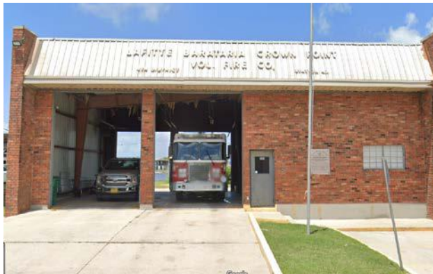
Image #4: Station 43 located at 5510 Jean Lafitte Boulevard in Lafitte
